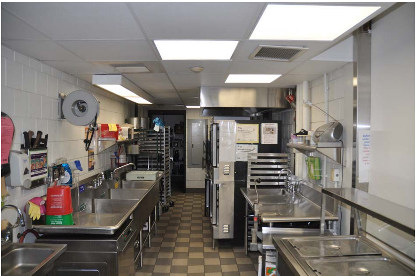
Picture 7.33 Under-sized Brooks kitchen
