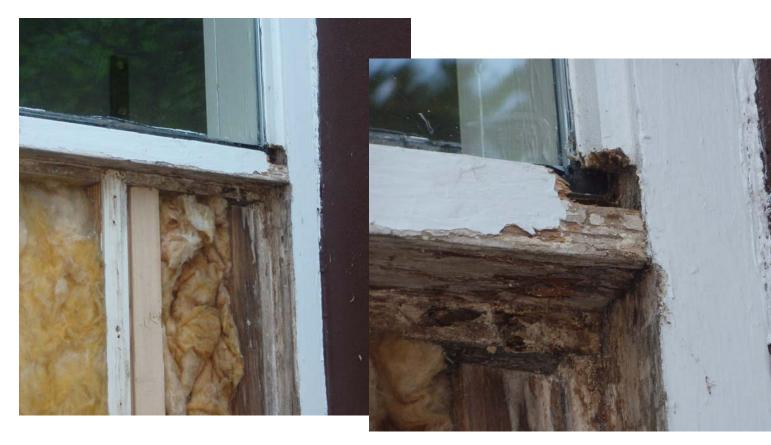
Facing the immediate need for repair, the district will replace this portion of the curtain wall with a metal framed wall containing an energy efficient window, instead of wood framing. This reactive approach, replacing sections of the curtain wall in a piecemeal fashion, is not cost-effective. We decided to revive the FY10 Hartwell Curtain Wall project in an effort to get out ahead of the problem.
