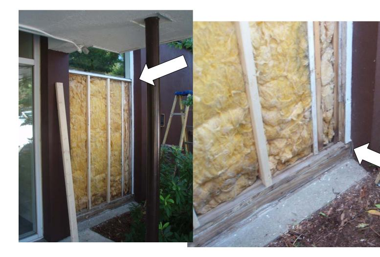
What we thought was a leak in the lower framing was actually caused by extensive rot in the sill at the bottom of the window, allowing water to leak down into the wall cavity and out into the room.
