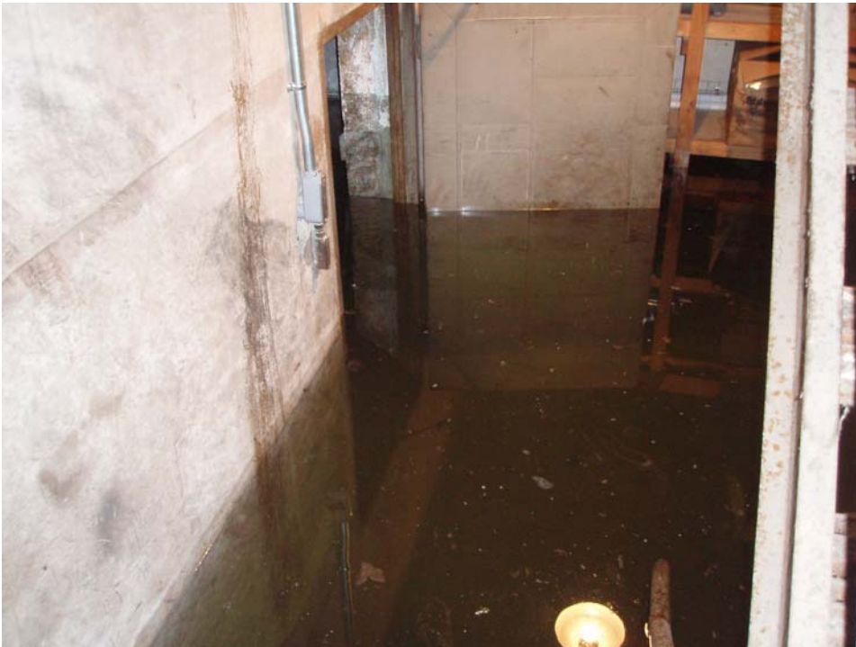
1. Smith Basement at 7:15 am
