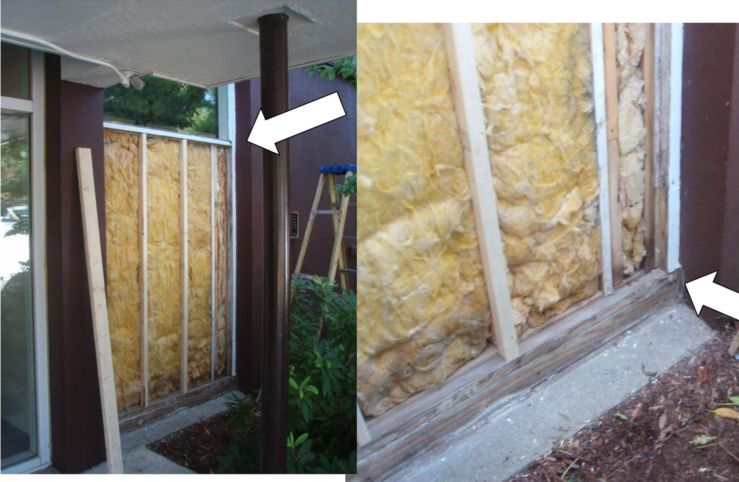
What we thought was a leak in the lower framing was actually caused by extensive rot in the sill at the bottom of the window, allowing water to leak down into the wall cavity and out into the room.
