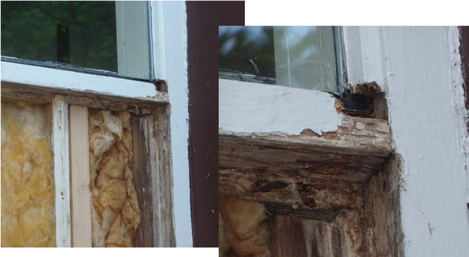
Facing the immediate need for repair, the district will replace this portion of the curtain wall with a metal framed wall containing an energy efficient window, instead of wood framing. This reactive approach, replacing sections of the curtain wall in a piecemeal fashion, is not cost-effective. We decided to revive the FY10 Hartwell Curtain Wall project in an effort to get out ahead of the problem.
