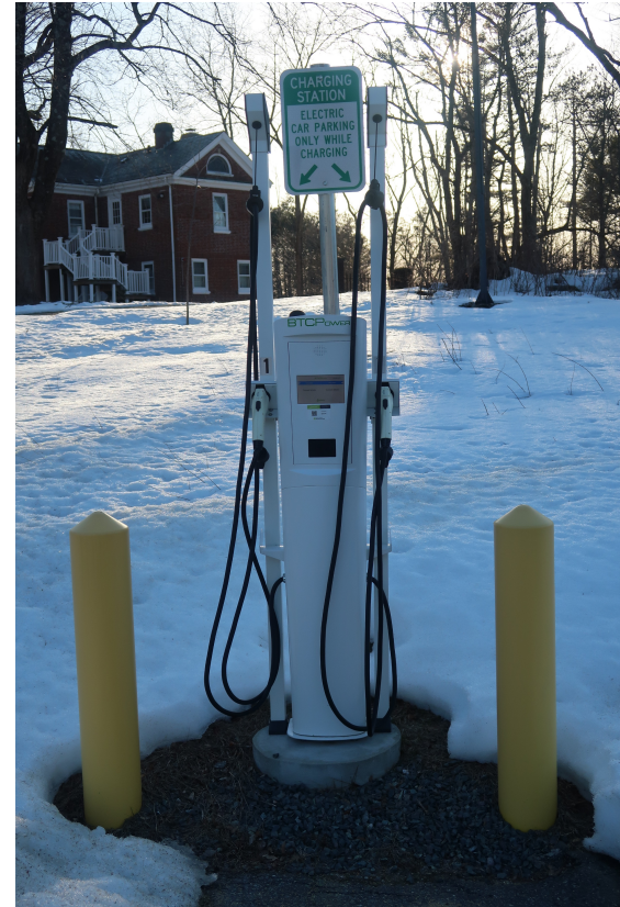
2-port Level 2 charging station with cable management system at Drumlin Farm
